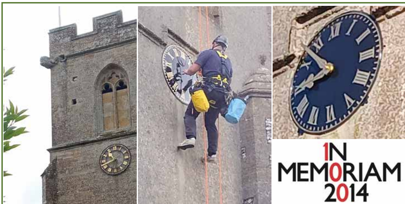
Above left: East Chinnock clock after work © East Chinnock Parish Council, 2025; Middle and Right: Works being undertaken on Baydon clock and after works © Baydon Parish Council, 2025
