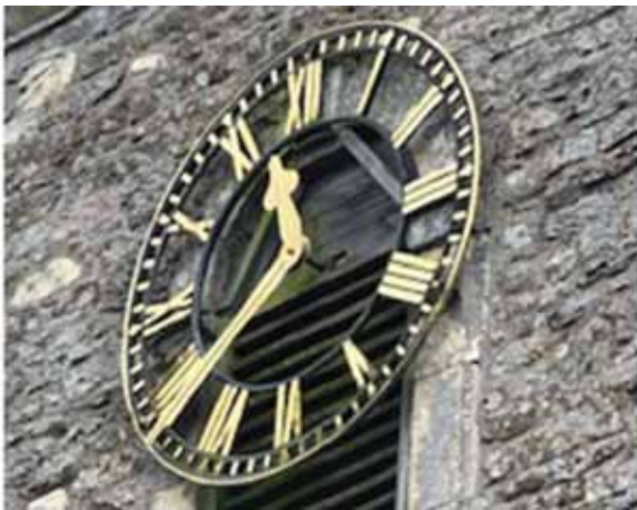
Top: the internal mechanism after work; Middle: church and clock faces before works; Bottom: face of clock after works (WM7455) © Glentham Parish Council, 2014, 2022 & 2023
