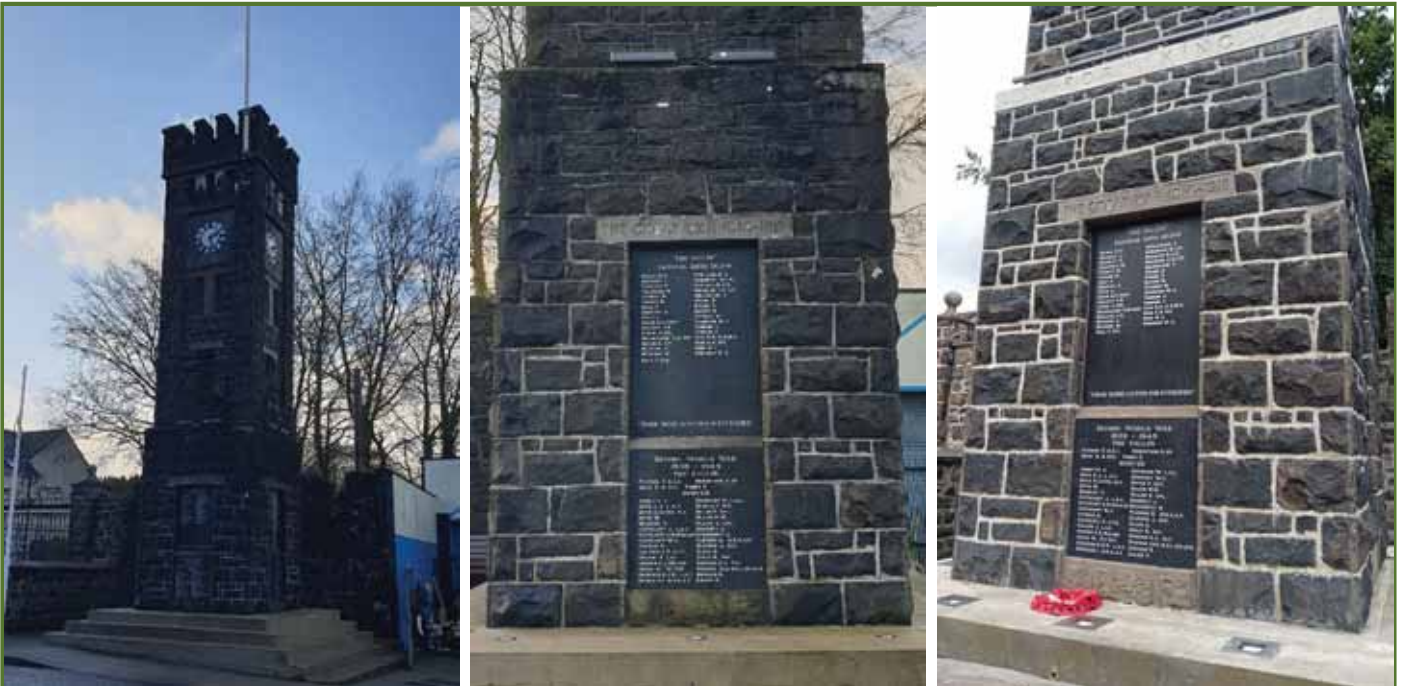
Above left and middle: Garvagh before works, and right: after works (WM11011) © Causeway Coast and Glens Borough Council, 2021 and 2022
