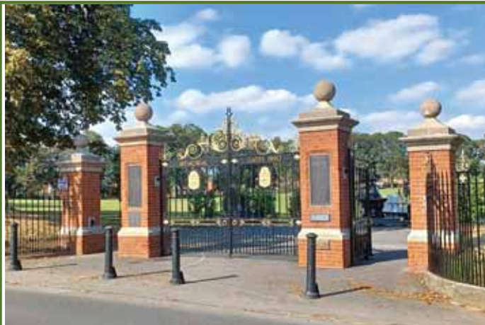
Above: Stowmarket memorial after works (WM8226); Below: Gates before and after work with plaques © Stowmarket Town Council, 2021
