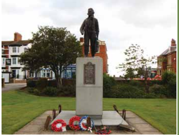
Above: RAF North Coates before works; Below, left to right, staining before works, applying SmartWater during works and the memorial after work (WM5955) © P Aitken, 2021
