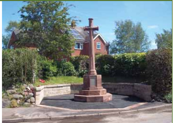
Above: Setting; Middle and below: Before and after works; All © M K Astley, 2020 and 2021
