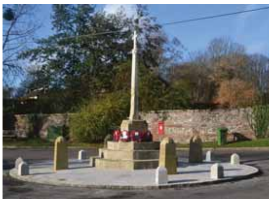
Over Wallop after works © Over Wallop Parish Council, 2020
