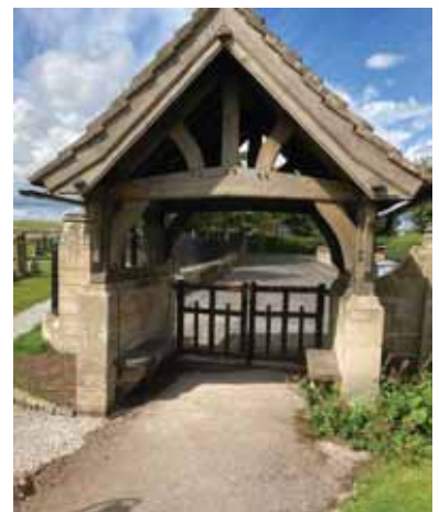
Marbury lychgate after works © St Michael's PCC, 2020
