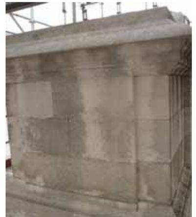
The top of the Cenotaph has the most severe staining
