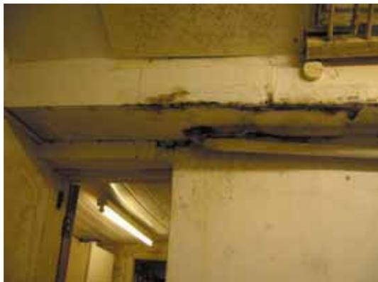
Internal damage by leaking roof © D Smith, 2013
