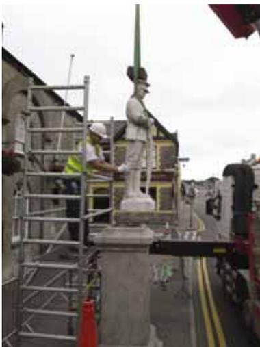
The soldier figure being carefully lifted from the plinth after being carefully strapped up © A. Davies, 2013
