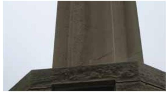
Before works showing split to the shaft of the war memorial and gap in the stone work caused by expansion of the metal supports © A. Williams, 2013
