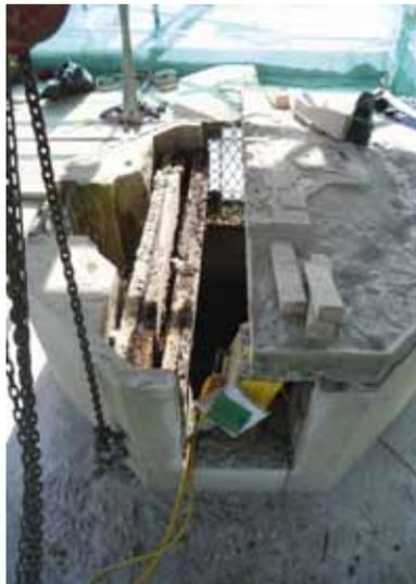
During works showing the heavily eroded metal supports inside the pedestal of the memorial © A. Williams, 2013
