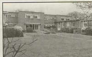
Oxted & Limpsfield war memorial hospital - threatened with demolition Photo courtesy of Cdr Josh Cosnett
