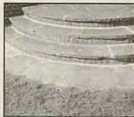
Repaired hard landscaping at Kemsing. Photo by Linda Drage
