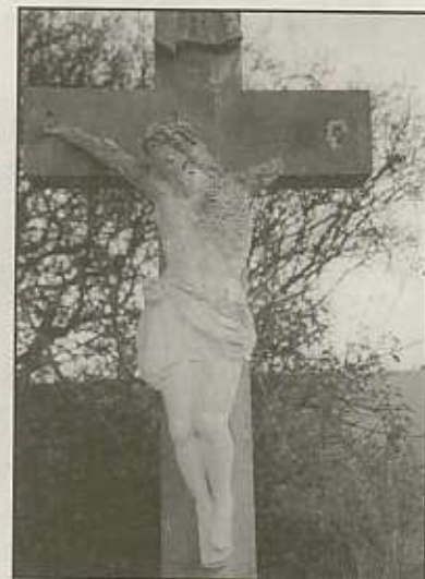
Damaged Christ figure at Tilbury juxta Clare, Essex (WWI) - repair work is now being considered. Photo by Maggie Goodall
