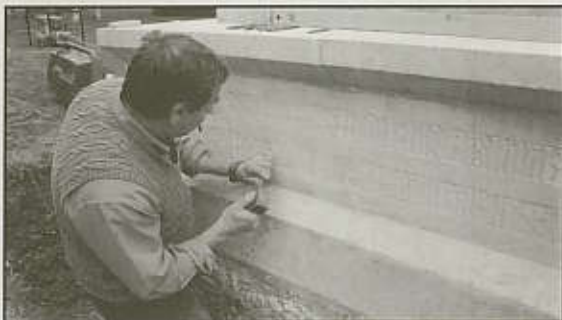
Using hand tools to sharpen the inscription on Barnes war memorial Photo courtesy of Gordon Newton of Burlite Ltd
