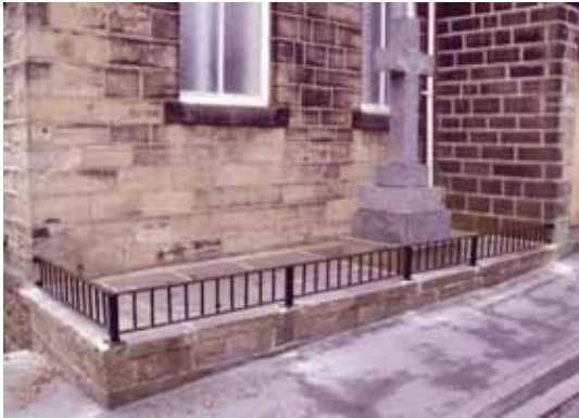
The newly installed railings around Exley Heath Methodist Church war memorial © Exley Heath Methodist Church
