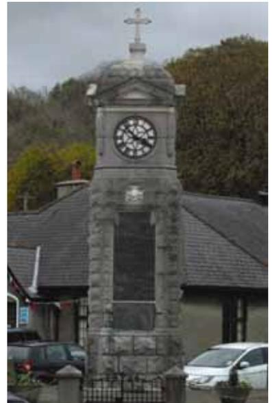
At Y Felinheli the combined grant funding of £8,760 supported repair and conservation works to the clock tower. This included scaffolding, raking out construction joints and re-pointing with lime mortar. The clock face was repaired whilst the timber was also treated. To protect the metal elements of the memorial SmartWater was applied as part of the [In Memoriam 2014](#) initiative discussed further on page 10.
