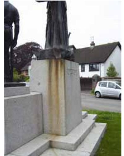
Staining caused by ferrous fixings within the structure © Cardiff Council, 2013
