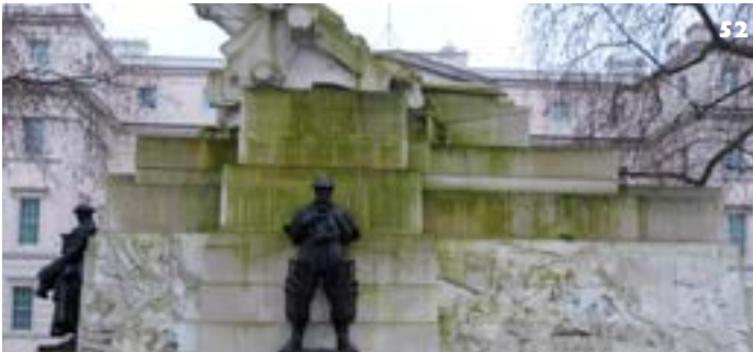
52: Algae will grow in any situation where there is a suitable combination of moisture, nutrients and environment. In the case of the Royal Artillery memorial at Hyde Park Corner, adjacent trees provide nutrients, while the poorly draining horizontal surfaces of the high level stonework are perpetually damp. © Odgers Conservation Consultants Ltd
