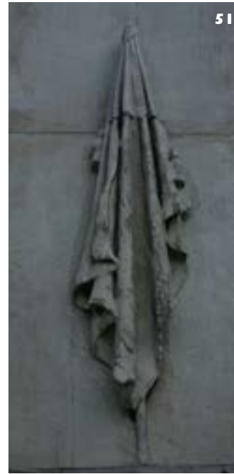
52: Algae will grow in any situation where there is a suitable combination of moisture, nutrients and environment. In the case of the Royal Artillery memorial at Hyde Park Corner, adjacent trees provide nutrients, while the poorly draining horizontal surfaces of the high level stonework are perpetually damp. © Odgers Conservation Consultants Ltd
