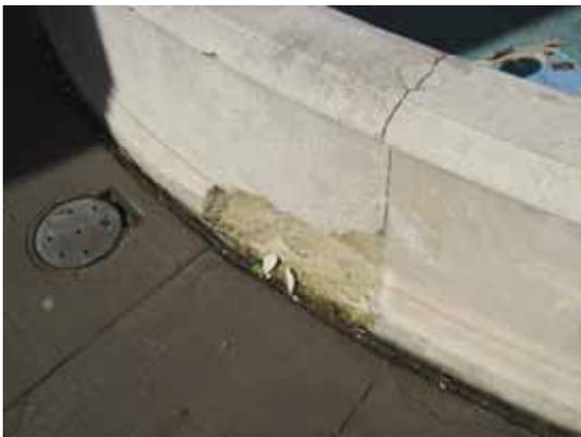
Base of the fountain, requiring an indent repair in order to prevent continued water ingress and degradation of the stonework © WMT, 2011
