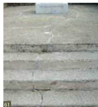
Fig 61 Concrete elements can be vulnerable to cracking, Craigie, Ayrshire © Craigie Community Council (2012).
