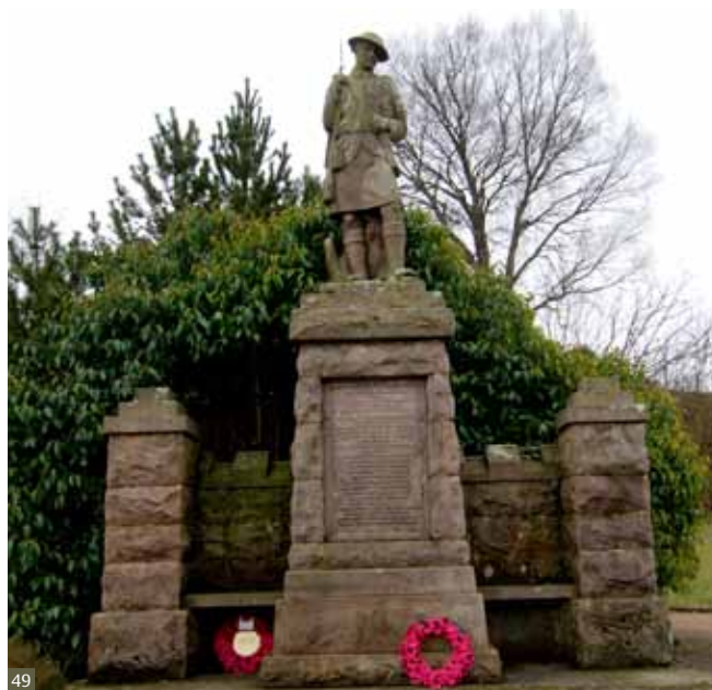
Fig 48 Plant growth shading can encourage damp conditions.
