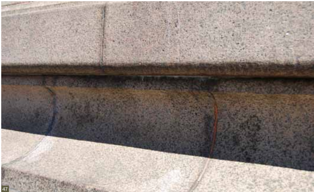
Fig 47 Abrasive cleaning can roughen the surface of polished or dressed masonry.
