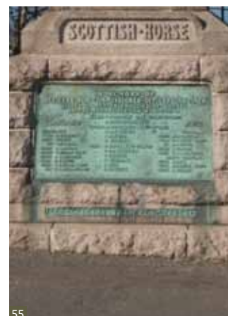
Fig 55 Staining caused by run off from bronze panel.
