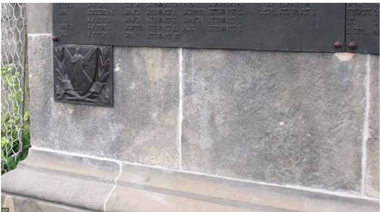
Fig 57 Fine joints re-pointed in lime mortar. Lossiemouth, Moray © George Wilson (2011).
