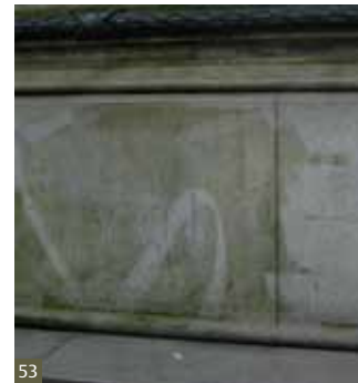
Fig 53 Uneven or aggressive cleaning can cause discolouration.
