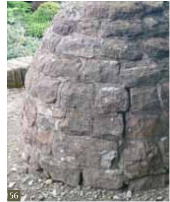
Fig 56 Defective pointing increases the risk of frost damage © Paul Goodwin (2012).
