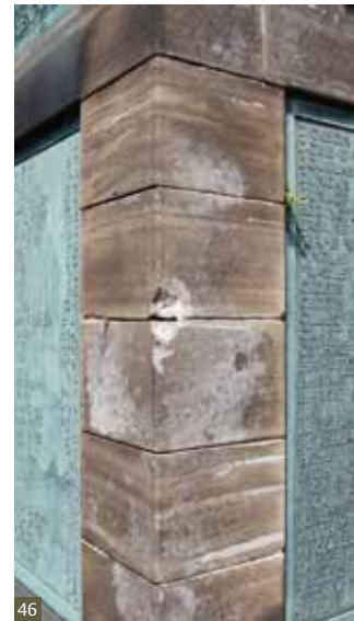
Fig 46 Impact damage to corner of ashlar masonry.
