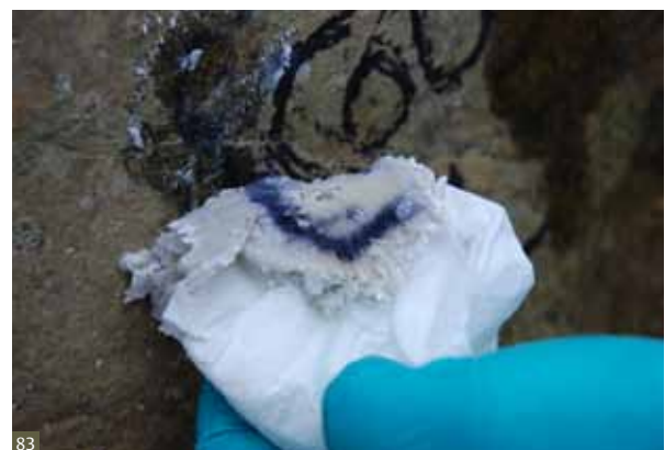
Fig 83 Using a poultice to remove graffiti.
