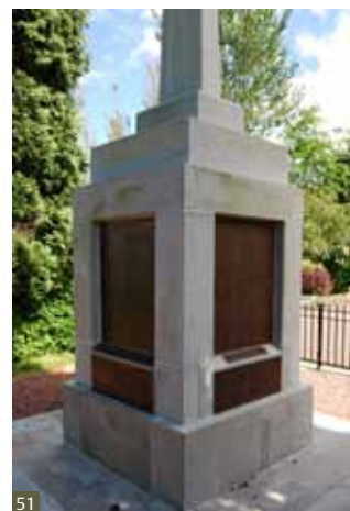
Fig 51 Bio-colonisation after cleaning.
