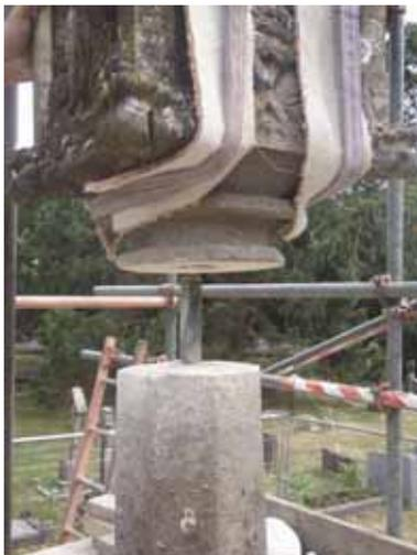
Taking the crown off the top of the cross reveals the copper dowel in need of replacement inside © Orchard Stonemasons, 2010
