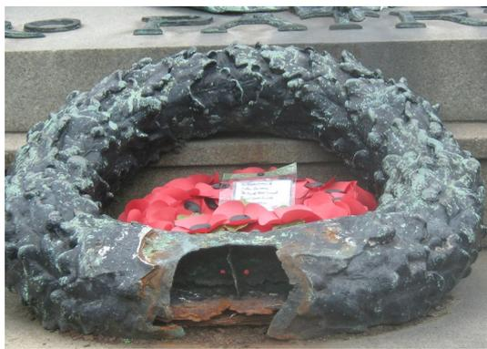
Untreated damage can speed up deterioration due to water ingress © War Memorials Trust, 2010
