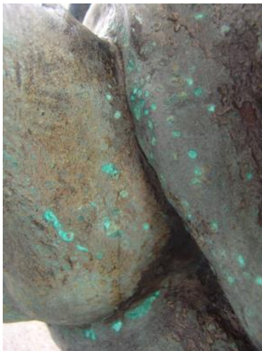
Active corrosion is typified by bright green pustules © Rupert Harris Conservation
