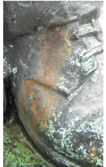
This staining has probably been caused by a rusting internal armature © War Memorials Trust, 2011
